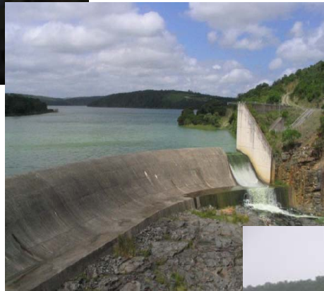
Bridle Drift Dam
