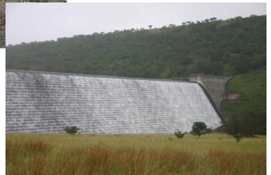
Wriggleswade Dam Spillway
